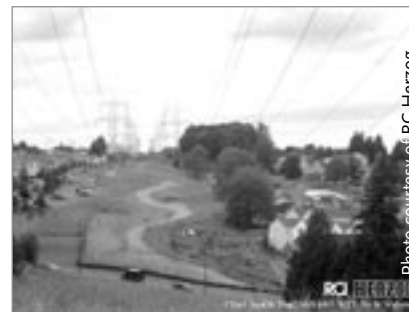
View of the progress on the new trail.
